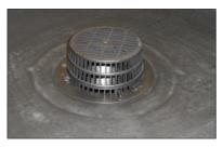
4) Install the leaf grate into the three locating tabs.
