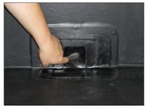
1) Install outlet into parapet wall before installing EPDM membrane. Install the ClassicBond EPDM membrane over the outlet with ClassicBond Bondina Adhesive. Cut the EPDM membrane away from outlet opening by 50mm. Apply ClassicBond Primer to the membrane, outlet face and into the outlet pipe.
