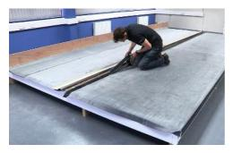
1) Fold the top sheet back to expose the seam area. Using a scrubbing pad apply the ClassicBond Primer to the seam area. Apply the primer past the seam edge to the line. ClassicBond Primer must be dry before application of PS tapes.
