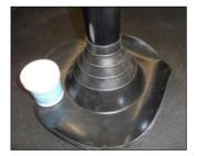
1) Cut the ClassicBond PS Pipe Seal above the raised "rib" one size smaller than the pipe diameter. DO NOT CUT THROUGH THE RIB. Pull pipe seal over pipe until base flange is in contact with the ClassicBond EPDM membrane.
