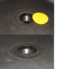
2) Remove the circular section of membrane and the yellow protective cap from the outlet.
