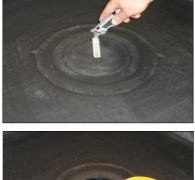
1) Fit the outlet into the roof before installing the membrane; ensure the outlet has the yellow protective cap installed. Install the ClassicBond EPDM membrane to the roof and over the outlet, place cutting guide over the pin and cut round the circular plate.
