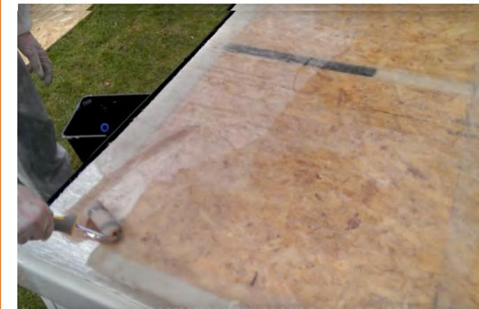
3) We suggest using 1kg on the deck and 0.2 or 0.5kg on the surface depending the matting type you have, after the resin has soaked you will start to see the boards . Proceed to step 4
