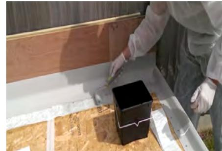
4) The kit will have a 75mm woven bandage or if you prefer cut strips of CSM and wet out with the resin allowing time to soak.
