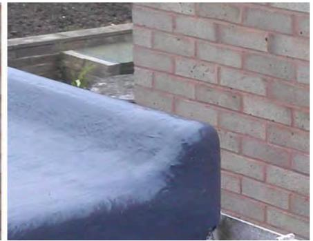
1) Cut the CSM approx. 150mm x 150mm double these up as 1 layer once stretched is to thin
