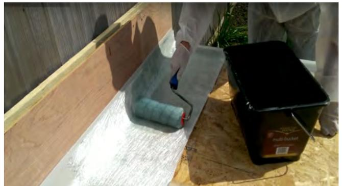
2) Mix approx. 2.5 to 5l of resin and start to wet the matting with the medium pile roller, This is easier with 2 people and the roller on a telescopic pole.
