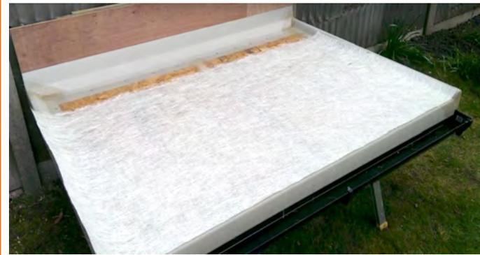
1) Cut the membrane FROM END TO END ideally following the fall of the roof this ensures any overlaps are falling in the direction of the water run off
