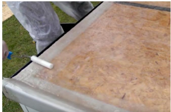
4) At this stage use the metal roller and consolidate the matting, your aim here is to draw resin to the surface, push the matting to the deck and remove all trapped air bubbles, the overall finish should be opaque, smooth and a nice wet film of resin on the top layer
